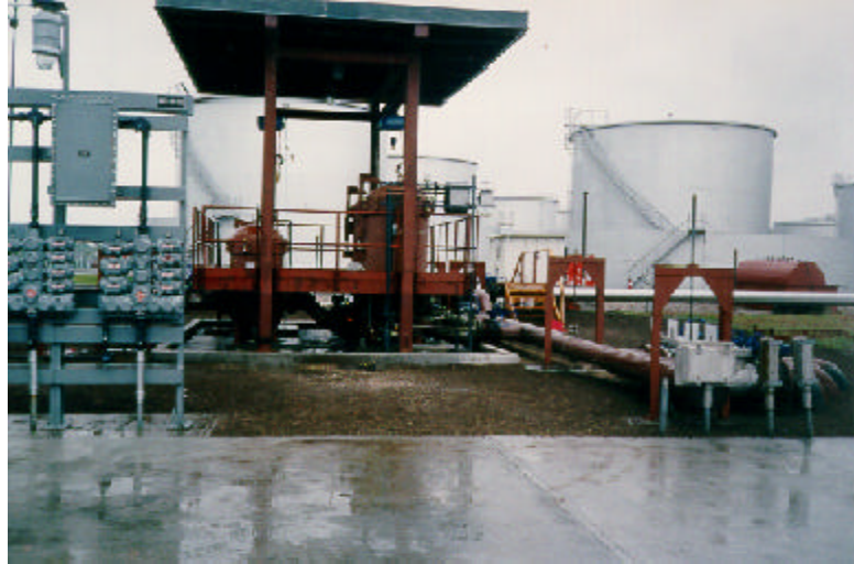
The JFK Airport fuel farm underwent reconstruction to achieve greater efficiency.
